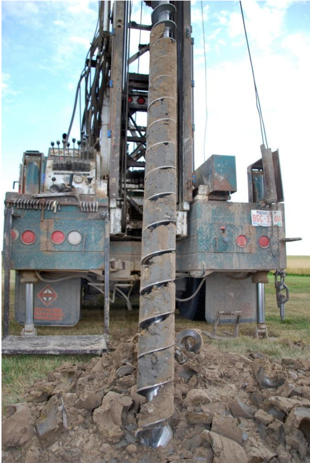
Plate 13. Glacial till encountered during drilling at piezometer nest 3.
